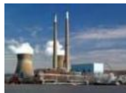
Thermal power plants
